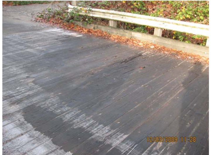
Sixth Street Bridge decking before repairs
