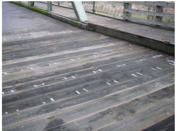
Sixth Street Bridge decking after repairs
